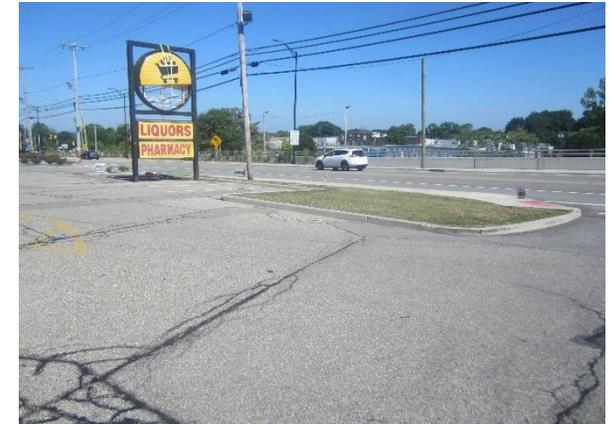
Stormwater is currently directed to an existing detention basin. Parking spots in the center of the parking lot to the north as well as the row of spots on the northeast corner can be replaced with porous asphalt to capture and infiltrate stormwater. A preliminary soil assessment suggests that the soils have suitable drainage characteristics for green infrastructure.
