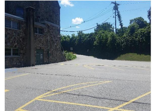
Stormwater is currently directed to the creek to the north that is downhill from the site. Parking spots on the north side of the parking lot can be replaced with porous asphalt to capture and infiltrate stormwater. A preliminary soil assessment suggests that more soil testing would be required before determining the soil's suitability for green infrastructure.
