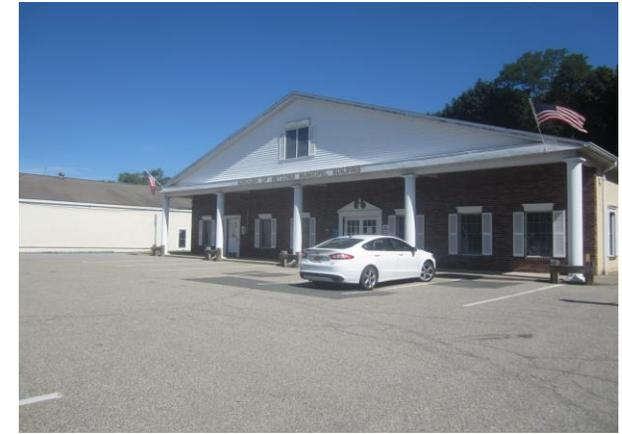
Stormwater is currently directed to an existing detention basin. Planter boxes can be attached to the downspouts on the eastern side of the building, two on each corner and two on the downspout at the center of the wall. Parking spots to the south of the building can be replaced with porous asphalt to capture and infiltrate stormwater. A preliminary soil assessment suggests that the soils have suitable drainage characteristics for green infrastructure.
